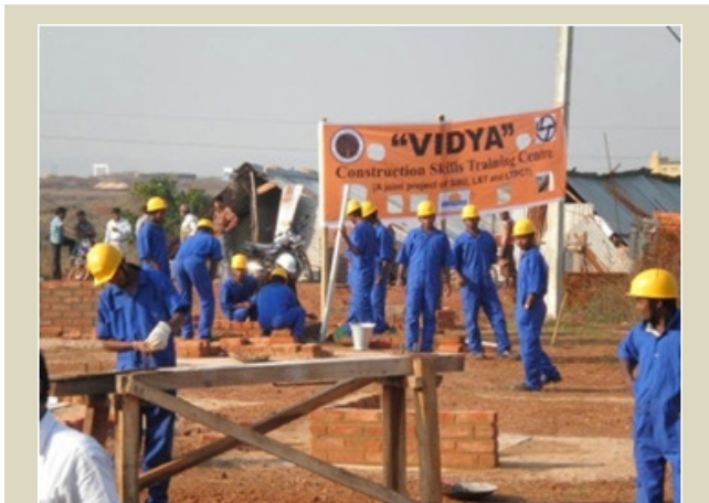
Training in Masonry
